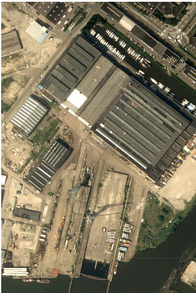
Aerial photograph of the NDSM wharf, Stichting Kinetisch Noord
