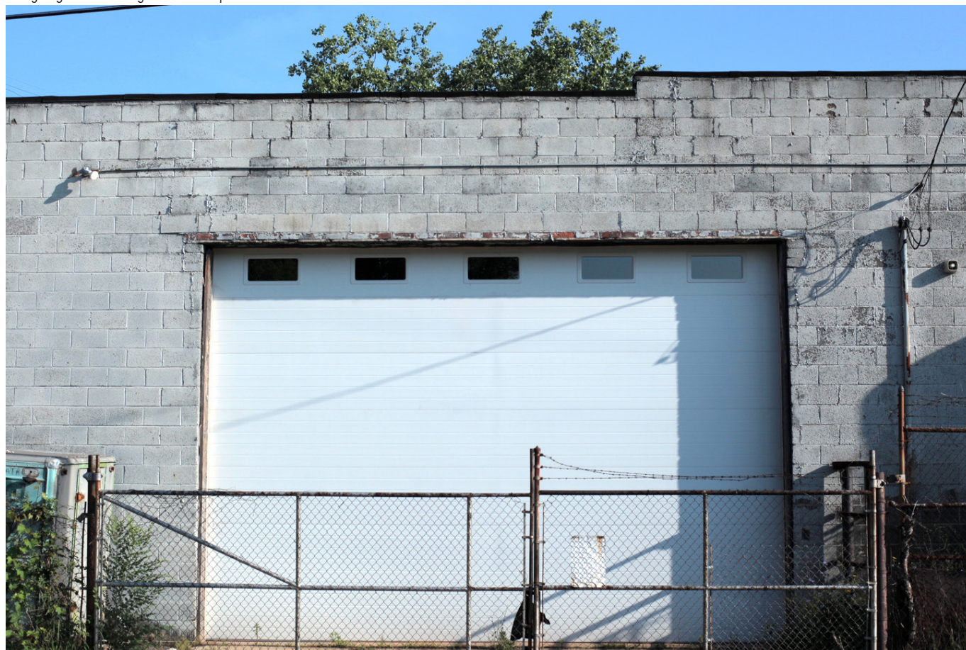
The garage door leading to the workspace.
