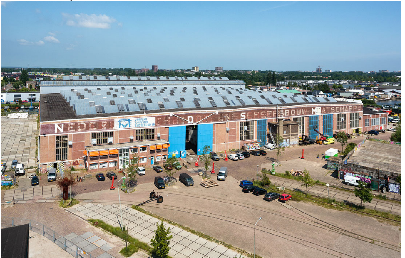
Exterior view of the main hangar. Photo: Ronald Tilleman
